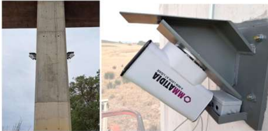
Figure 7: Installation of the LDVs under the viaduct
