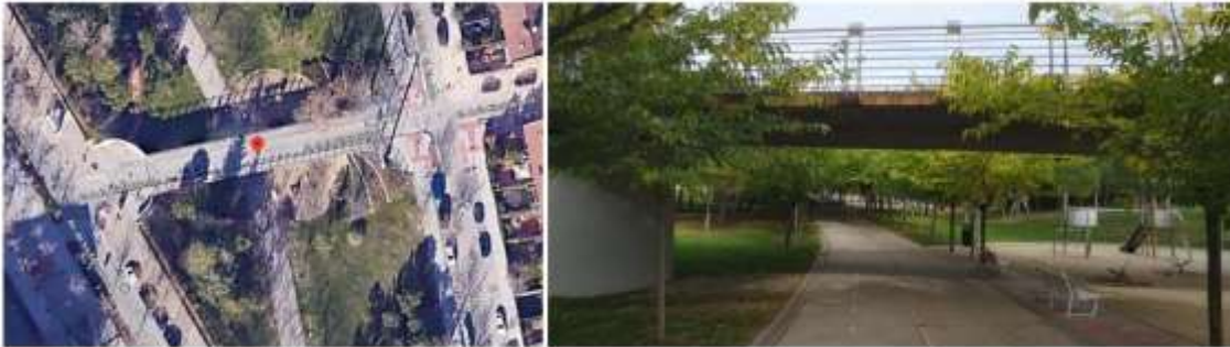
Figure 12: Google Maps view (left) and image of the bridge(right)
