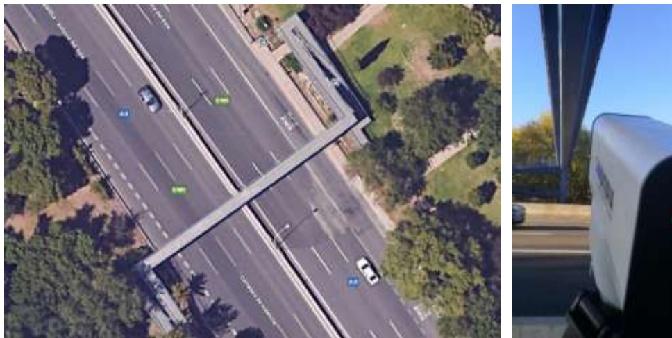
Figure 1: Position of the laser vibrometer under the walkway.
